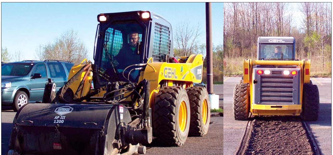
When the Universal open drum was lowered into the asphalt, it proceeded to mill through the full 4 in. of asphalt and base to a 6-in. depth, leaving behind a smooth layer of grindings. After viewing the Universal demo, the other vendors declined to plane.
